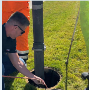
Vacuum removal of debris
