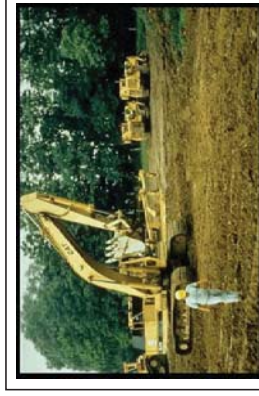
Fig. 14. The severely compacted soil of a temporary construction yard used daily by heavy equipment for four months, shown before deep ripping, topsoil replacement, and decompaction.
